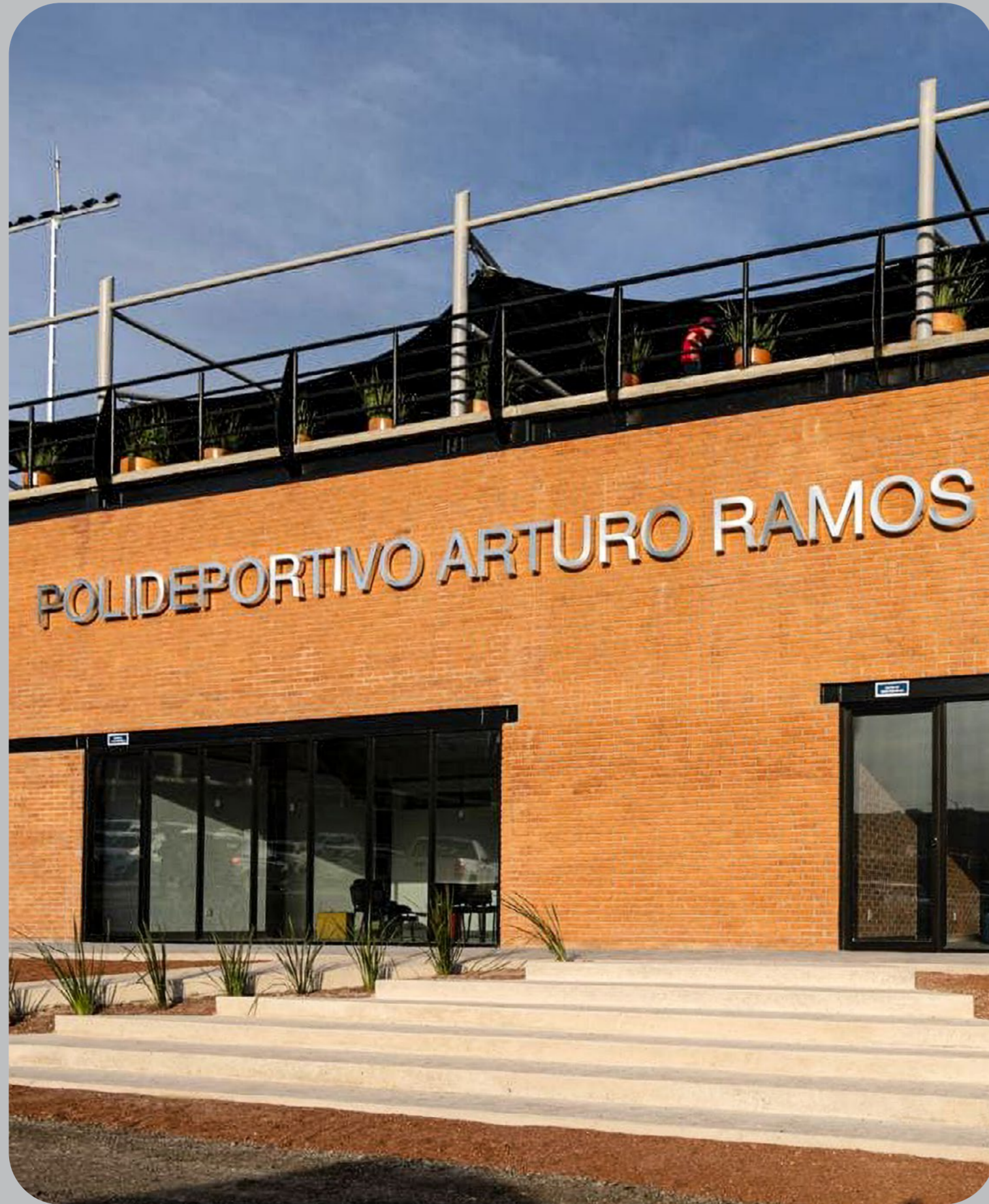
Peñamiller leads in the number of sports facilities per 10,000 inhabitants with 38 sites, followed by Arroyo Seco with 26 and Colón with 17.
